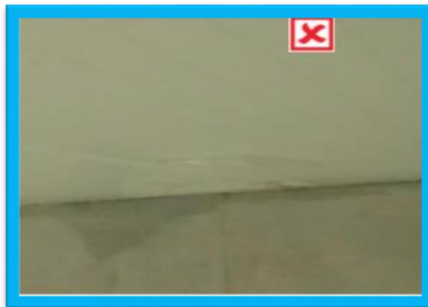
Figure 10: Water seepage / leakage on the wall / floor
