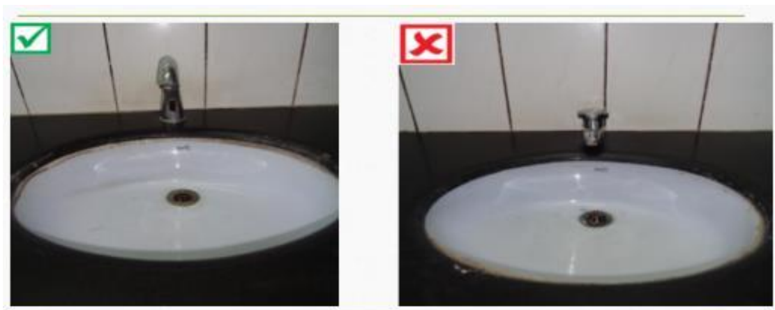
Figure 33: Touch free (hands free) taps at wash basins to avoid cross contamination
